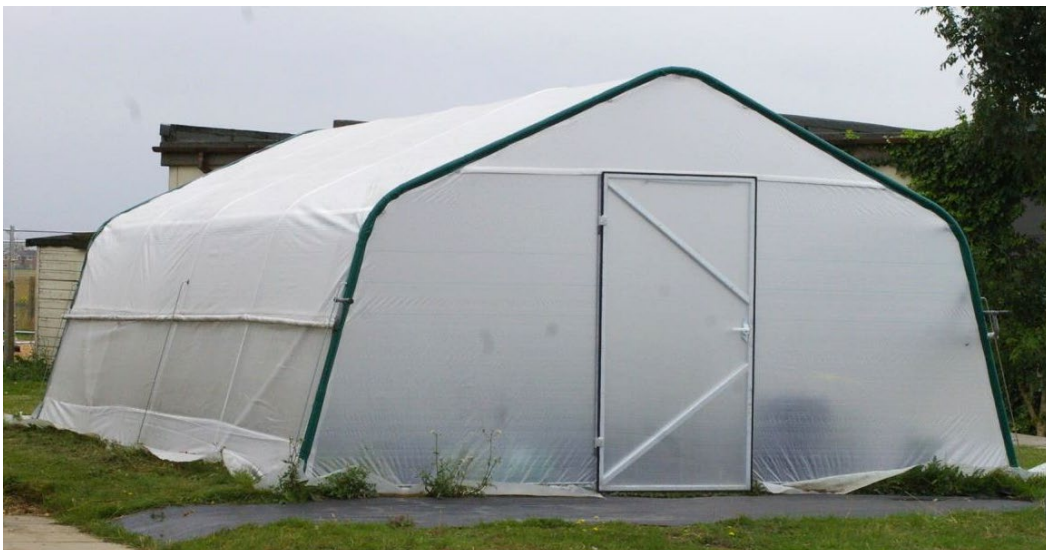
Figure 1 - Garden polytunnel (Haygrove Ltd) used to conduct the deficit irrigation trial.
